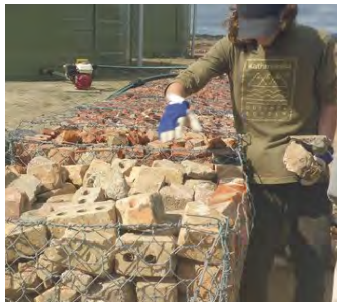
Forktree Hill Project: Building a gabion retaining wall from salvaged building rubble
